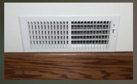
**PRO TIP:** Un-screw vent caps and clean them out thoroughly, removing dust and dirt to help air flow easily.
